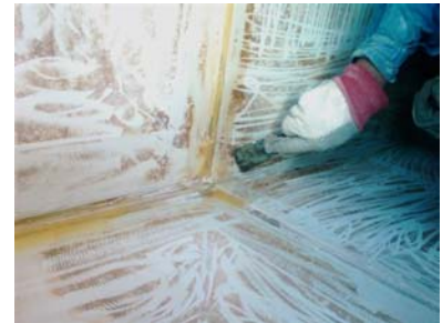
SolarSeal was used to seal joints between panels
