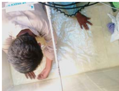
Application of the SolarTech Sheet Laminate
