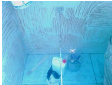
Preparation of the surface
