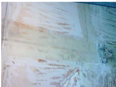
Joints are sealed by single layer stripe of SolarTech Sheet Laminate
