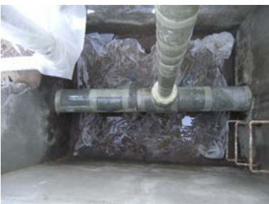
Pipe after SolarTech material application
