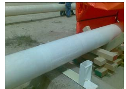
Finished application with white SolarCoat as a top layer
