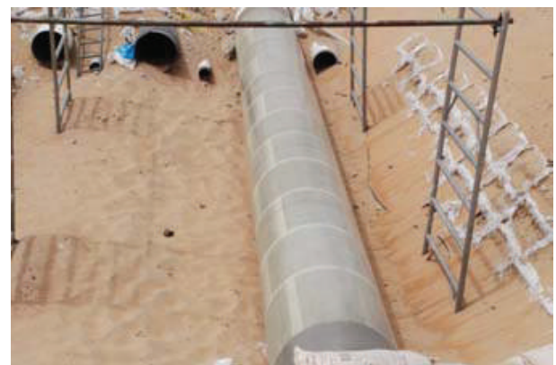
Pipe after the repair
