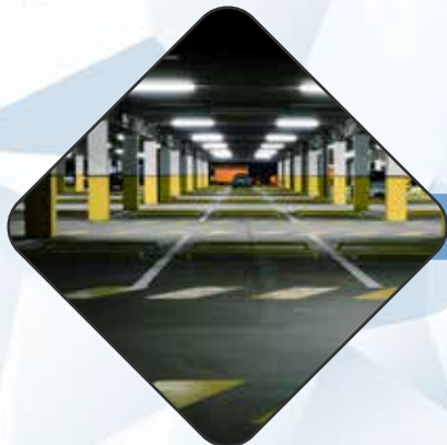
Underground parking structures
